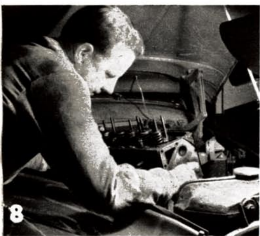
If the water pump is to be removed it is best done before the head is lifted. Space is limited. Ensure that your grip is firm.
